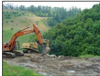
Stable, but highly compacted, reclaimed areas support grasses and shrubs, and often little else. Preparing the surfaces for trees requires excavating rooting zones with a backhoe ( left ) or ripping the surface ( right ). Both methods loosen the rooting zone for better seedling survivability and tree growth.
